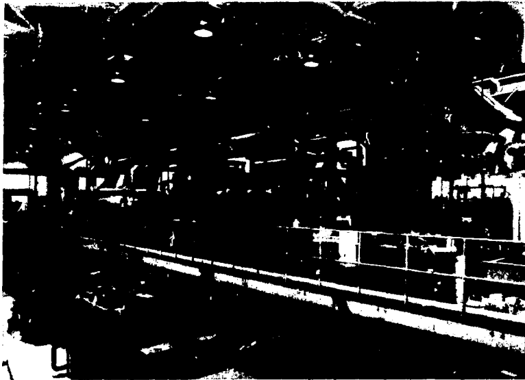
Figure I.7. Interior view of the cryogenic wing. The ends of the five cold boxes of the refrigerator are barely discernible behind the cryogenic piping.
